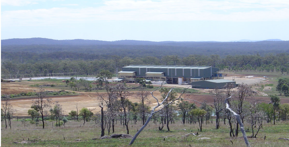
Figure 2: The Goondicum Processing Plant
